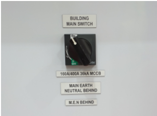
Main Switch is suitable for 320A/400A .
